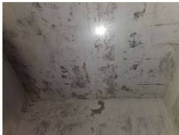
Picture 3. Moistness of the reinforced concrete slab and walls.
