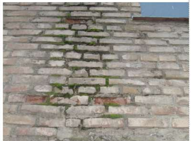
Picture 4. Damages of moisturized brick and mixture under the influence of temperature
