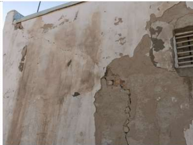
Picture 1. Cracks in the walls as a result of uneven building sinking
