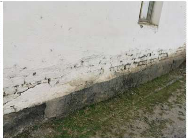
Picture 2. Moistness of the building's foundation and basement
