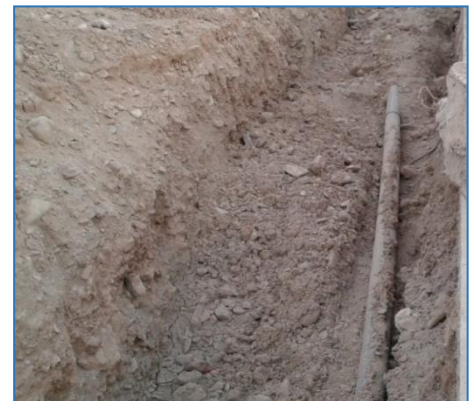
Figure 3. The state of failure of the trench connecting the main pumping station of the Sherabad cement plant with the water well №5 due to landslides. F_{t,d} - Possible external deformation forces.
