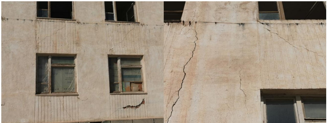
Picture 1. Cracks formed in the outer wall as a result of uneven deformation of the building.
