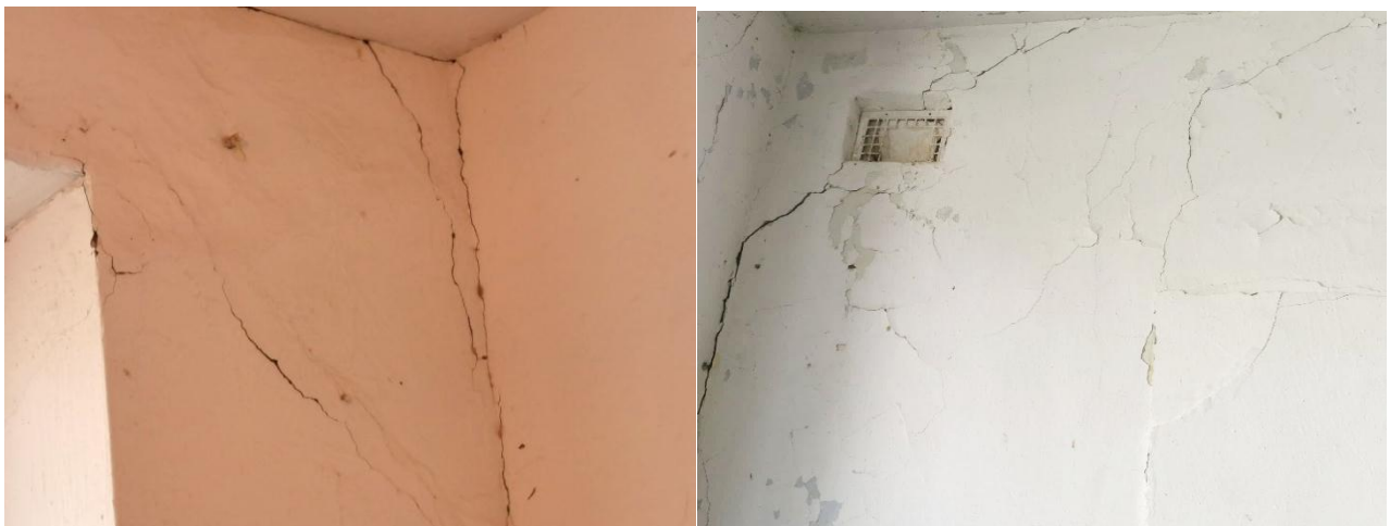
Figure 3. The outer and inner walls are cracks formed at the junction node.
