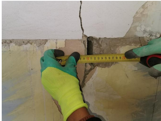
Picture 2. Measurement of the width of the cracks formed in the outer wall as a result of uneven deformation of the building.
